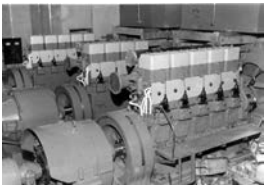
Diesel generator at the Tokyo Astronomical Observatory Norikuradake Corona Observation Station
